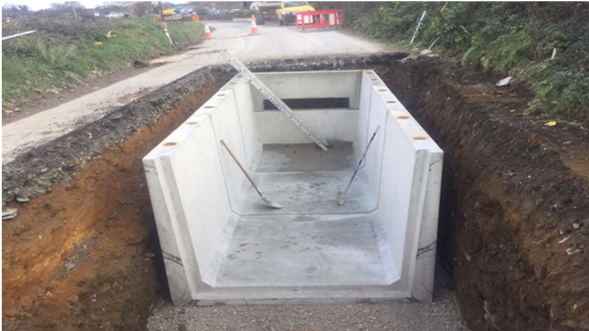
Image 1.3: Example of a Joint Bay During Construction
