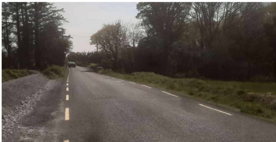
Image 1.7: Example of a Reinstated Road Following the Laying of Underground Cables
